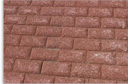
*Figure 14: Brick-stamped concrete*
