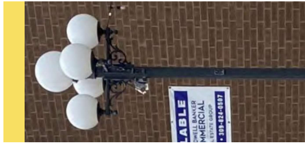
Existing globe light fixture.
