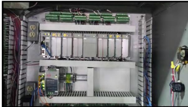
*Existing Bristol Babcock RTU – components were made up of electronic card CPUs and power supply regulators*
